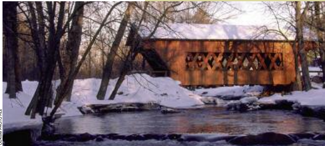
BELOW: SAXEVILLE COVERED BRIDGE.
