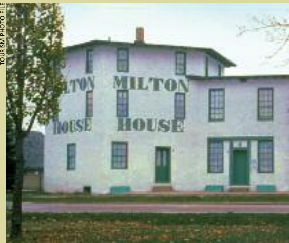
BELOW LEFT: LINCOLN-TALLMAN HOUSE IN JANESVILLE. LOWER RIGHT: BELOIT RIVERFRONT. RIGHT: MILTON HOUSE MUSEUM.
