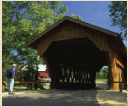
Saxeville Covered Bridge.
