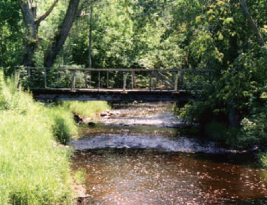
Along Rustic Road 82, Fond du Lac County.
